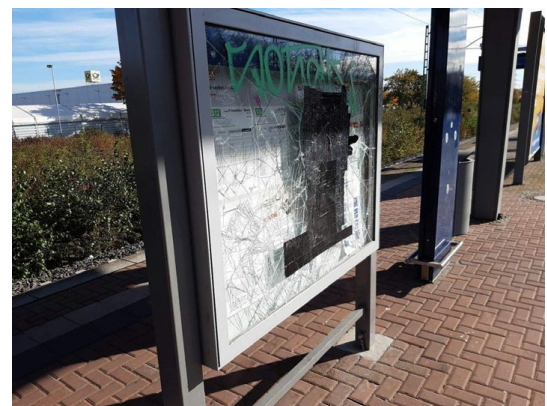
Vandalismus in Köln Airport-Businesspark
